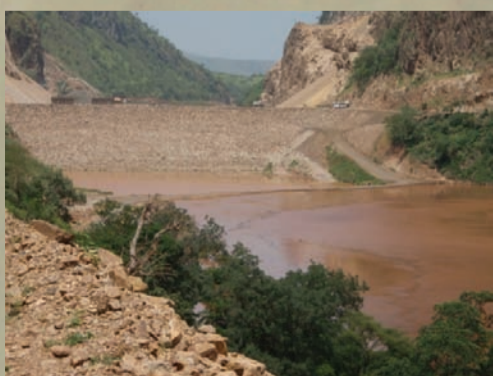
(fig.4. Upstream Cofferdam)
