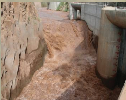
(fig.3. The Omo River flow diverted through the three tunnels)
