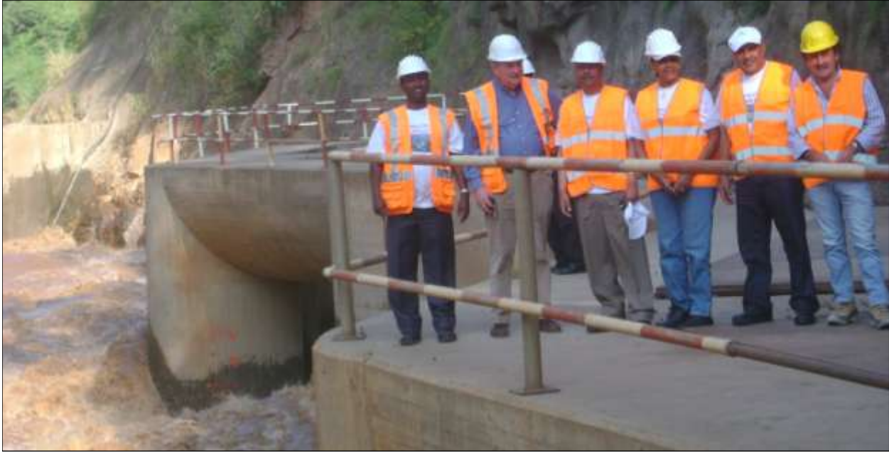
Visit at the three Diversion Tunnels' inlet area
