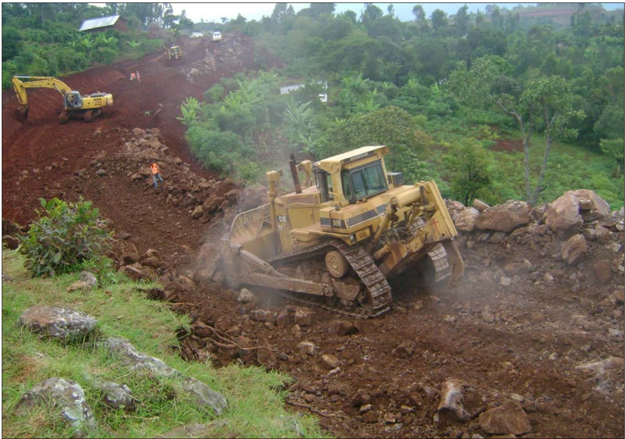
The realigned Chida-Sodo Road construction is progressing well, Welayta
