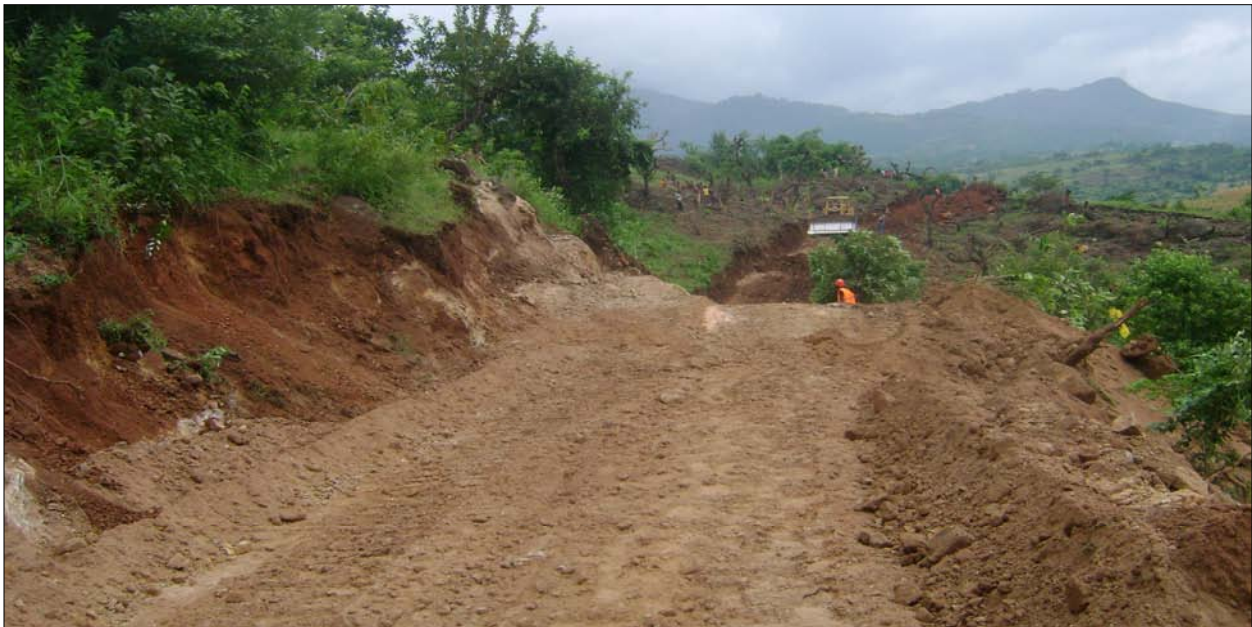
Chida-Sodo Road Construction
